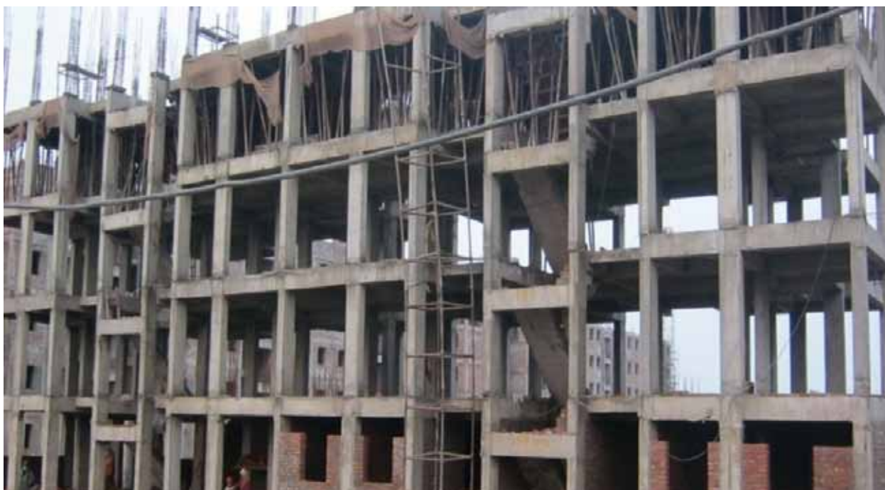
Construction of Tower No. 5 at Bhalaswa Jahangirpuri
