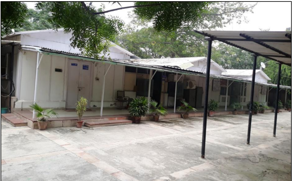
Renovation of Office Building at Raja Garden.
