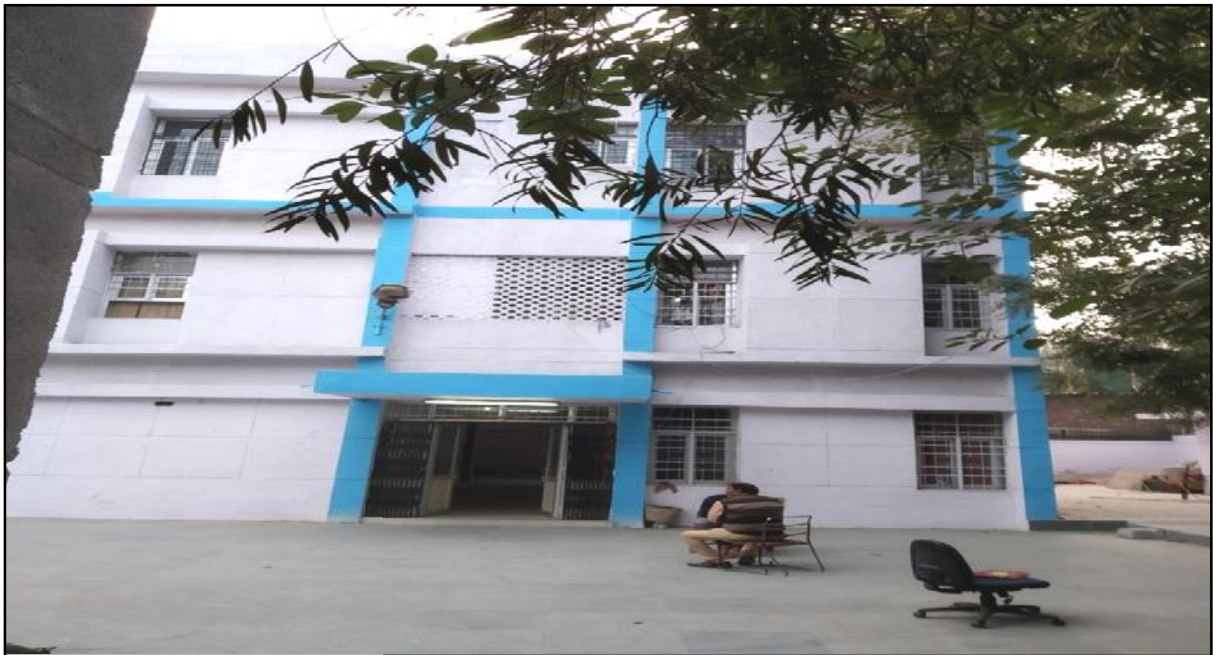
Upgraded Community Hall at Pillanji
