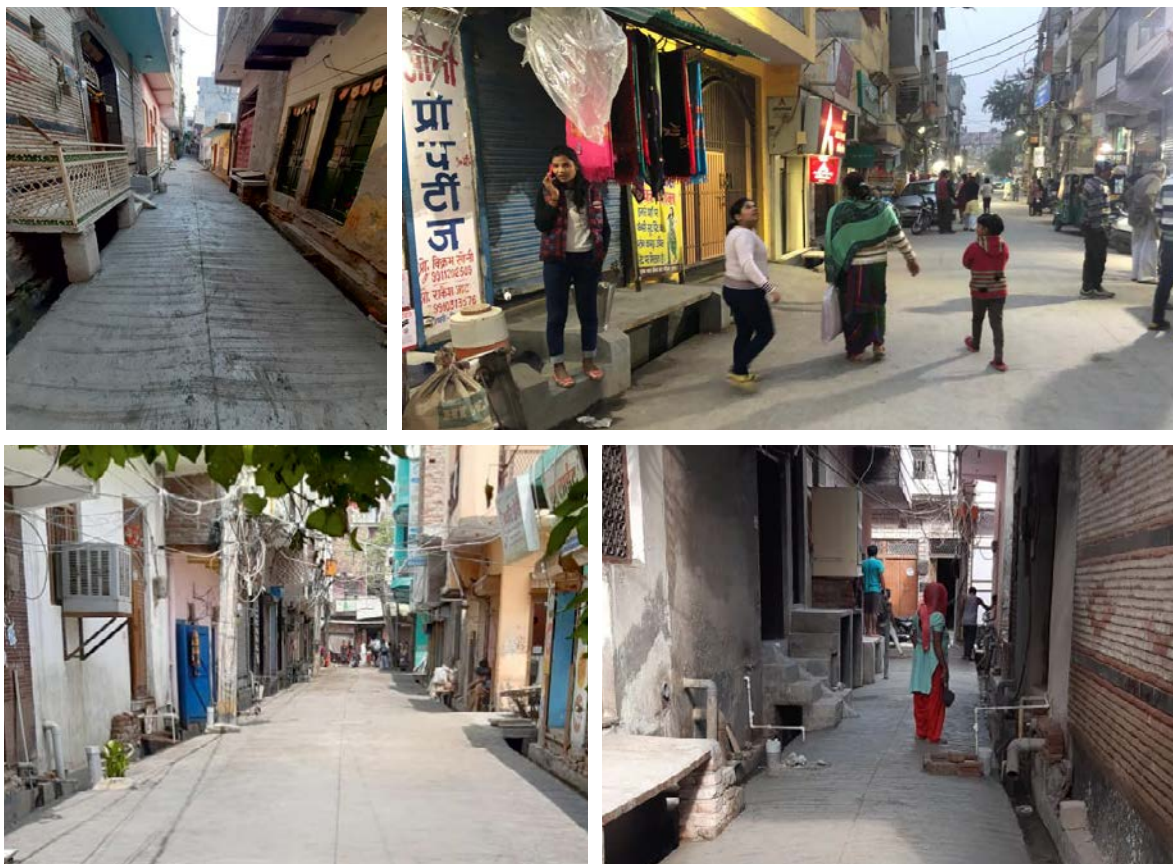
TYADB: C/O road and drain at Mangal Bazar road, Amar Colony, Gokalpur.
